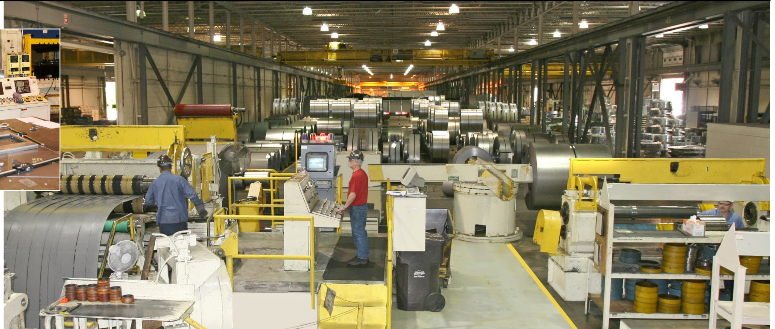
The Dennen Steel Service Center can slit up to 72" master coils. Slit coils are banded then staged for stamping at the rear of the facility, or moved to bays for JIT delivery or storage.
